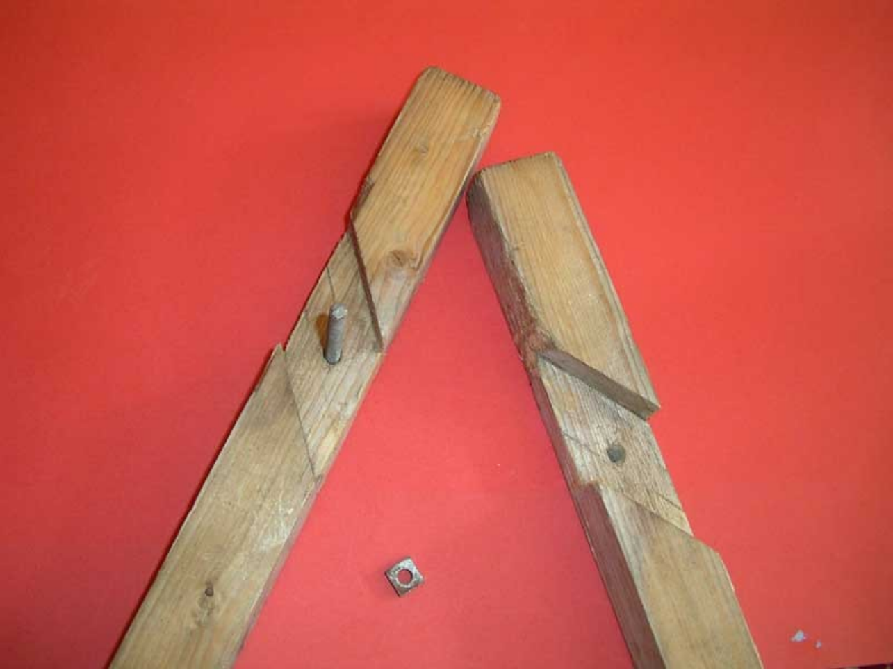
Close up of the joint
